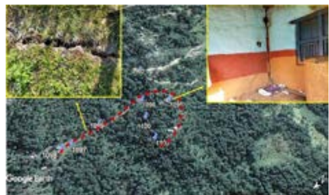
Figure 8: Google earth image of Gaurete (Banskharka) showing instability with observation points where the red dotted line shows cracks observed in the area.
