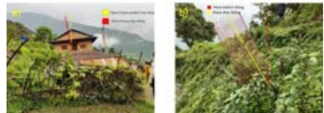
Figure 9: Tilting of a) house and b) tree.
