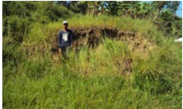
Photo 6: Land subsidence by more than 1m.
