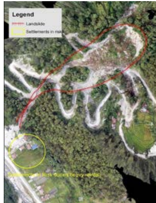
Figure 11: Orthomosaic image of Deopur showing slope failure and settlements in risk during heavy rainfall.
