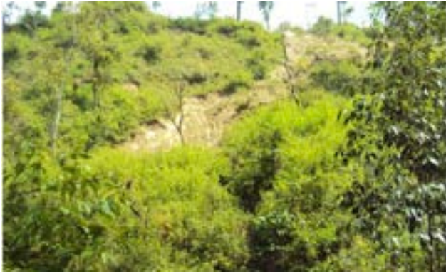
Photo 1: Mass movement alongwith development of and cracks and creeps in the sloppy terrain
