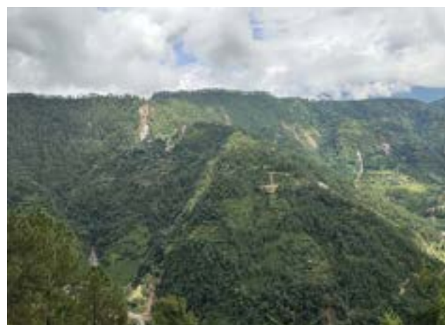
Figure 10: Series of Landslide observed from Isma at Musikot area.
