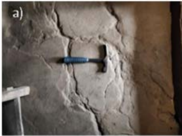
Figure 4: Observed cracks and sinkhole: a) filled cracks in the ground floor and b) sinkhole in cultivated land
