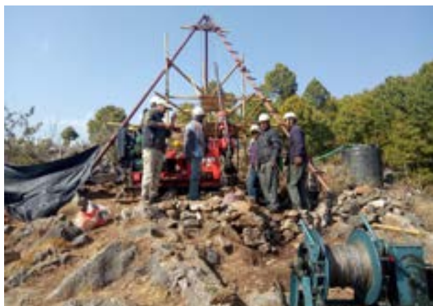
Photograph 2: Set up for drilling work at site
