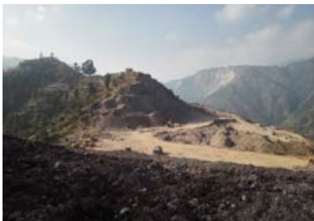
Photo 4: Maruti cement Kakurthakur
