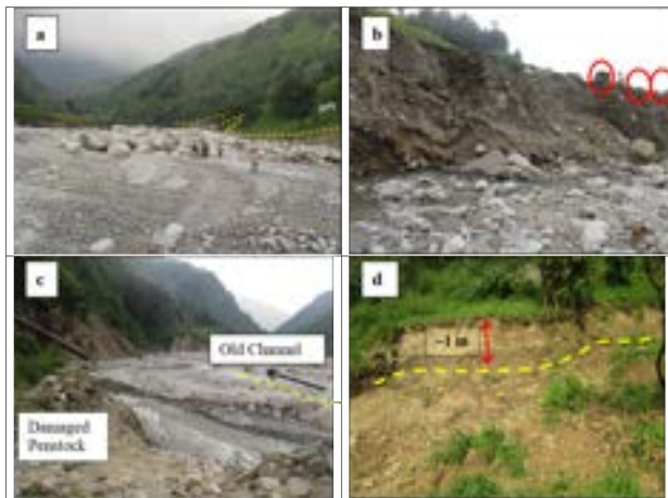
Figure 12: a) Boulders deposited by flood on the Kailash Khola (view of upstream from destroyed Shaini Bazar); b) Bank cutting on unconsolidated alluvial soil, and houses(abandoned) at risk; c) Channel shifting leading to bank cutting and damage of a Hydro power at Shaini Bazar; d) Scar of reactivated colluvial soil slide above Shainigaun.
