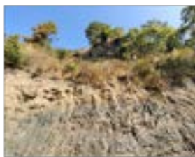
Plate- 8. Contact between Slate and carbonate member Benighat Slate
