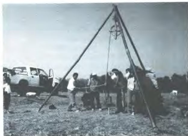
Fig. 2: Performing Standard Penetration Test (SPT) in the field.
