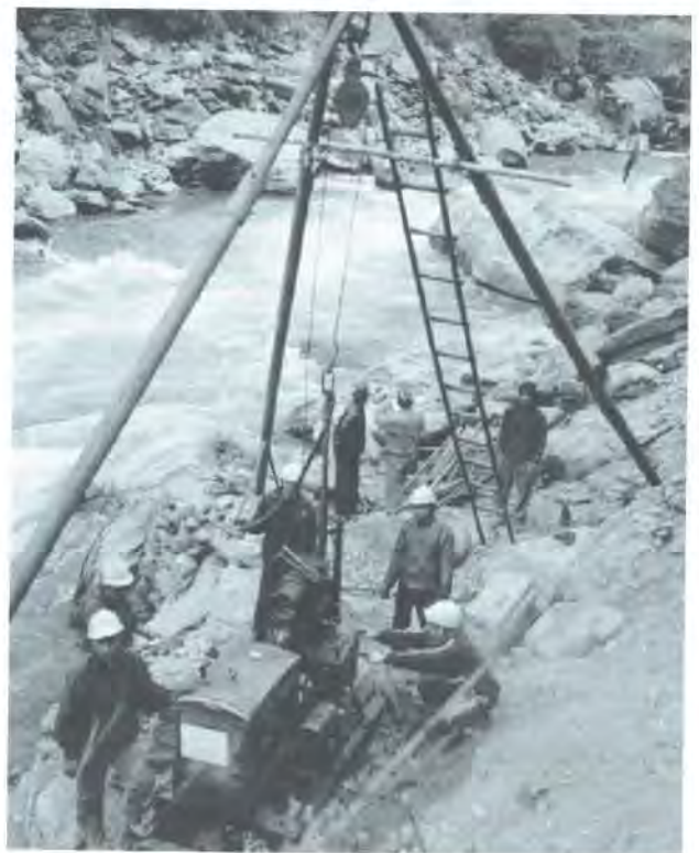
Fig. 5. Drilling of borehole BHN K0+220 LA1 aside the Bhotekoshi River
