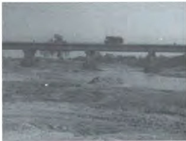
Fig. 10. Illegal sand mining from the right bank in Budhi Khola bridge
