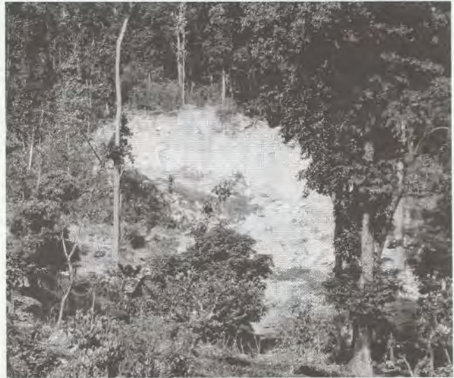
Photo 13 Landslide on the right bank of Jhupra khola
