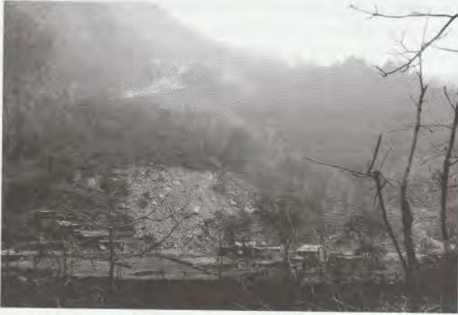
Photo: 1 Big landslide in Ratopani village on the Beni-Jomsome road which swept away many houses
