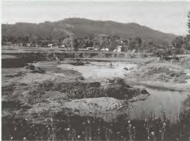
Photo 15 River bank cutting near Jitpur (Khorke Khola)
