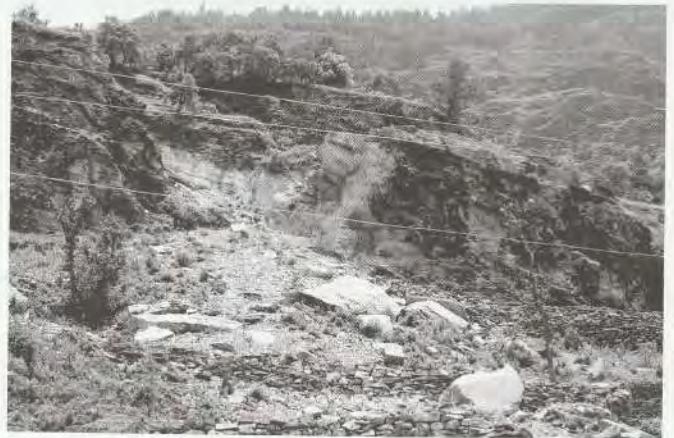
Photo: 4 Landslides on top of the Aul village threatening the people
