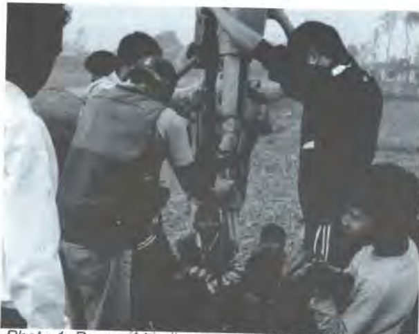
Photo 1: Power driven auguring in the soil to investigate sub-surface geology
