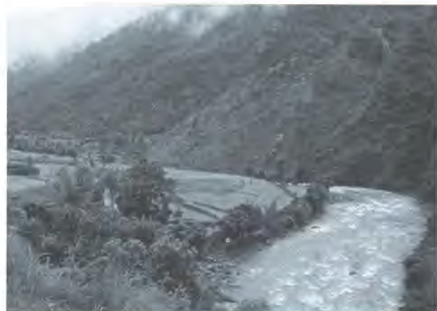
Photo 2: Landslide at the left bank of Barigad River near Burtibang
