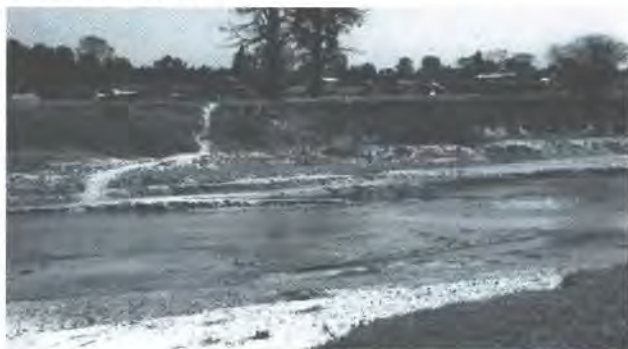
Photo 6: Houses are in risk from Bank cutting and flooding (Northeast of Siurajpur Village)
