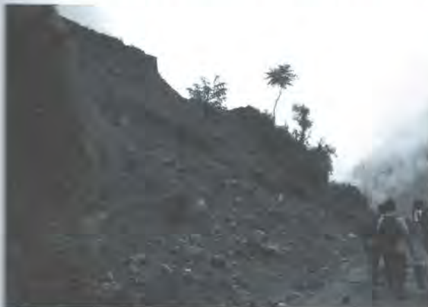
Photo 1: Road blocked by slide due to heavy rain on the way to Burtibang from Wami Taxar
