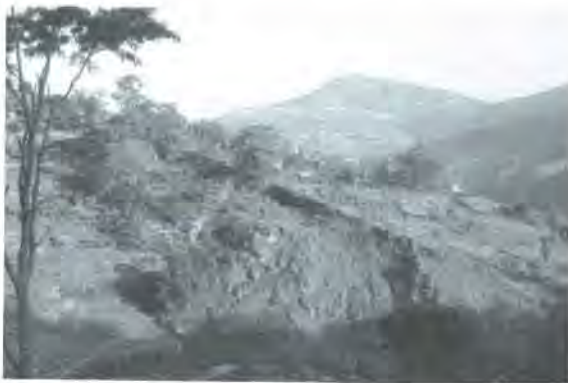
Fig. 2: Landslide at the Left bank of Kailash Khola.
