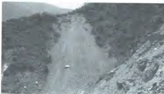
Fig. 3: Landslide due to road construction near Oli Gaon
