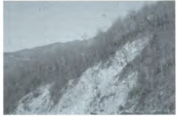
Photo 4: Landslide in purple shale at right bank of Chaira khola
