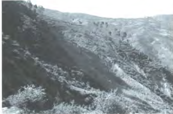
Photo 1: Big landslide in shale above Beraju village
