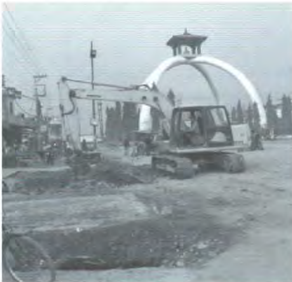
Fig. 20: Construction work for sewerage drain in Ramananda Chowk
