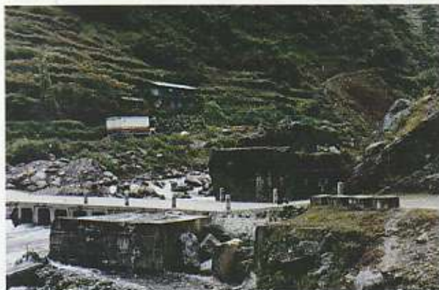
Larcha Cause way with remnants of previous bridge and police station.
