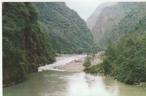
Debris flow is going to block Bhote Kosi River and damage the intake site of Bhote Kosi Hydro Power, power house.
