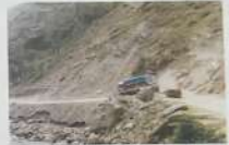
Landslide in Bhangra area
