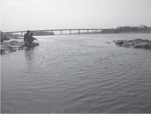
Figure 25: Bridge over Narayani River
