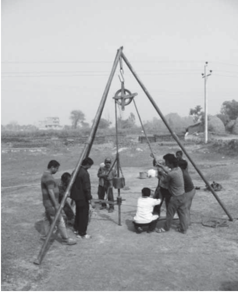
Fig. 2: Performing Standard Penetration Test(SPT).
