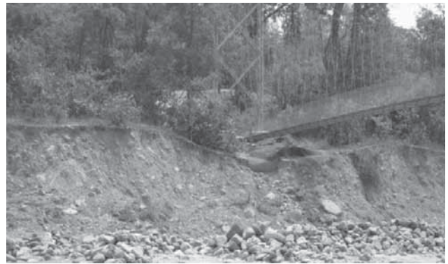
Fig. 18: Suspension bridge constructed in the northern part of Sukha Khola, near the forest is endangered due to river bank cutting.
