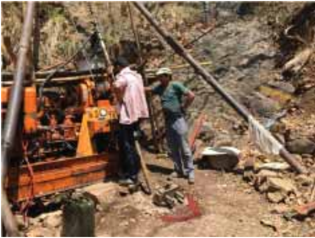
Drilling Work at Dhaubadi Iron Prospect, Dhaubadi, Nawalparasi
