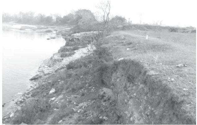
Fig. 14: Bank Cutting in right bank of Narayani River
