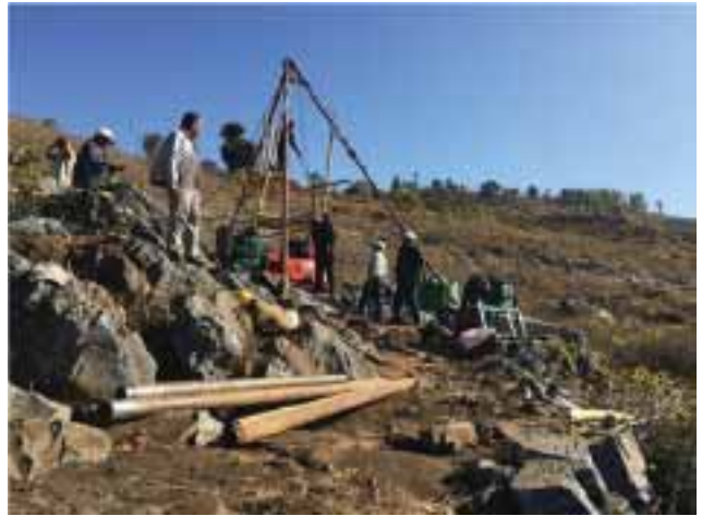
Drilling Work at Boje Limestone Prospect, Khotang
