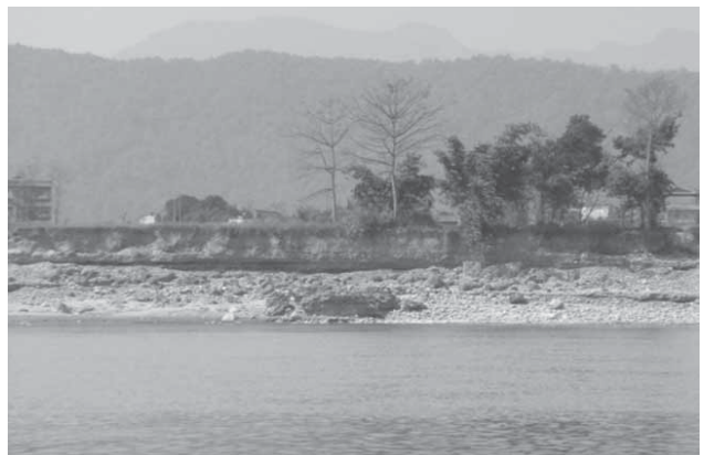
Fig. 16: Showing River bank cutting in left bank of Narayani River.
