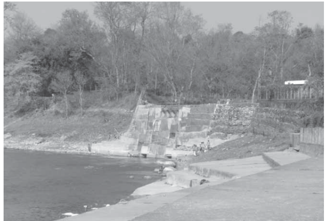
Fig. 15: Embrankment in Narayani River
