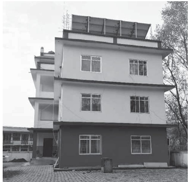
Fig. 7: Newly constructed building for data acquisition and analysis in Regional Seismological Center, Surkhet.
