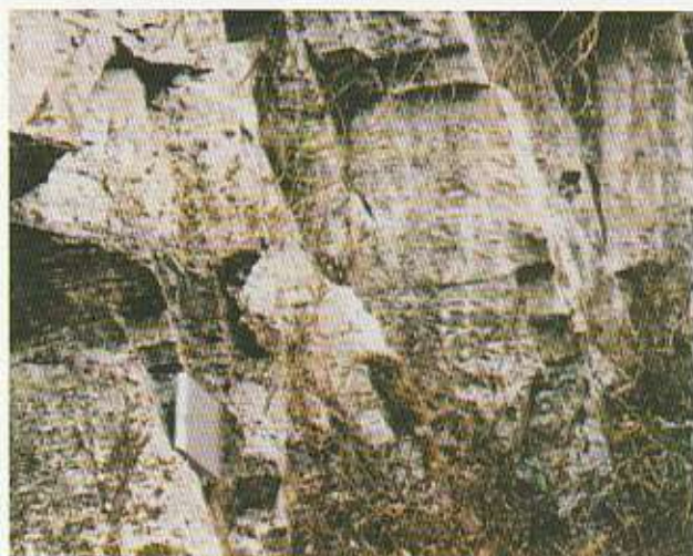
Photo 16: Highly jointed white gneiss at 101.75km.
