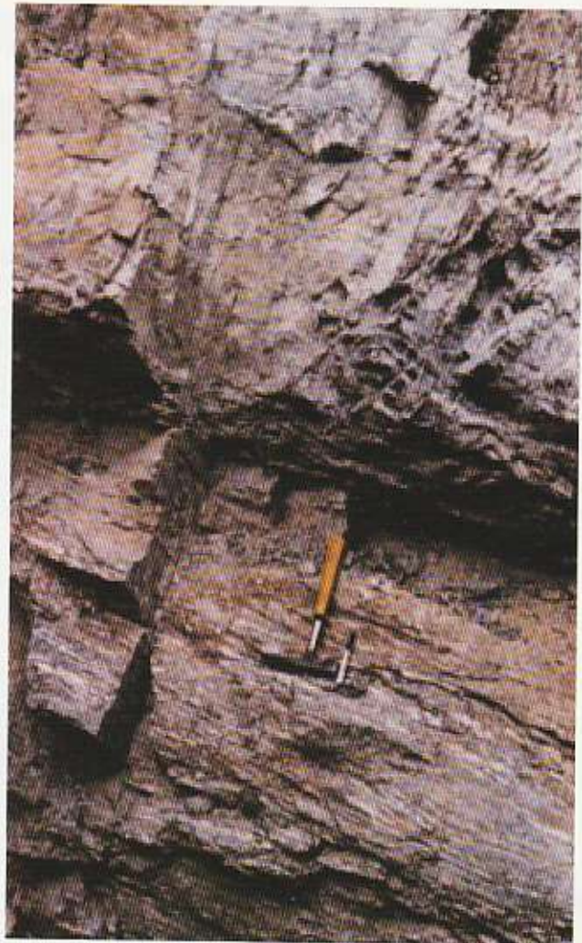
Photo 19: Block fall has caused hanging of upper part of the gneiss.
