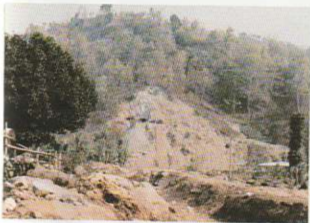
Photo 13-B: Tunnel leading to Mai Khola power house under construction.
