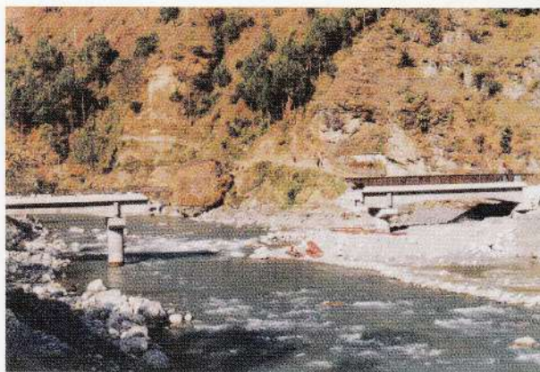
Photo 23A: Bridge over Kaligandaki River under construction.
