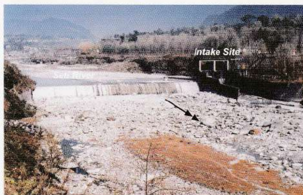
Photo 2: Seti dam and intake of Seti canal on left bank of Seti River.
