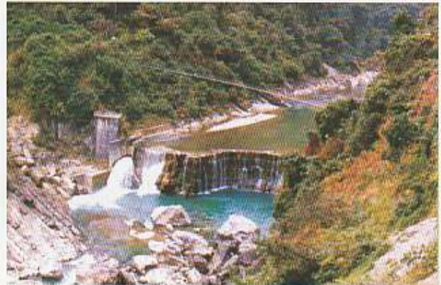
Photo 2: A hydro-electric power dam at 4km from Butwal.
